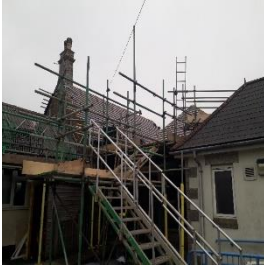
Full replacement of the pitched roof covering
