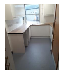
Lanner School Nursery kitchen refurbishment
